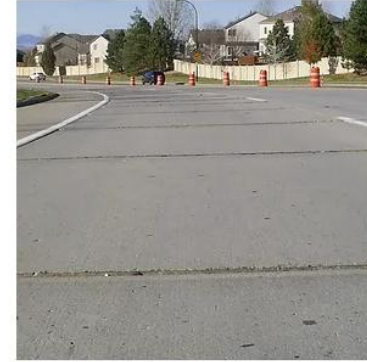
Faulted Joints
