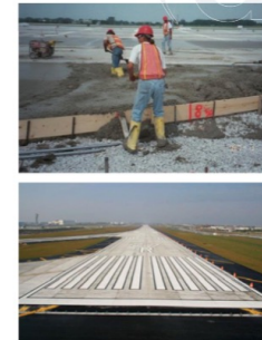
Fig. 5.1b—Concrete runway reinforced with 66 to 85 lb/yd 2 (39 to 50 kg/m 2 ) of steel fibers (O'Hare Airport runways, Chicago, IL).
